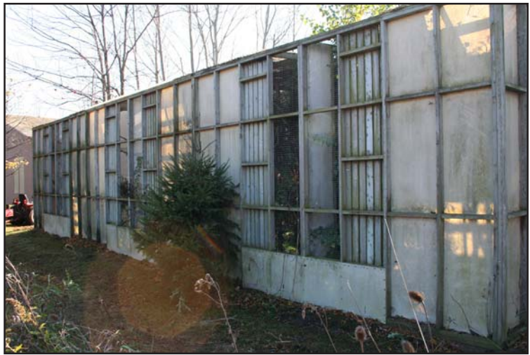
Short-eared complex before winter paneling installed
