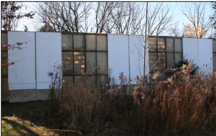
Short-eared complex after winter paneling installed
